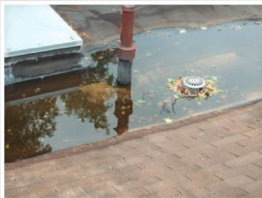
Ponding Water/Clogged Drain
